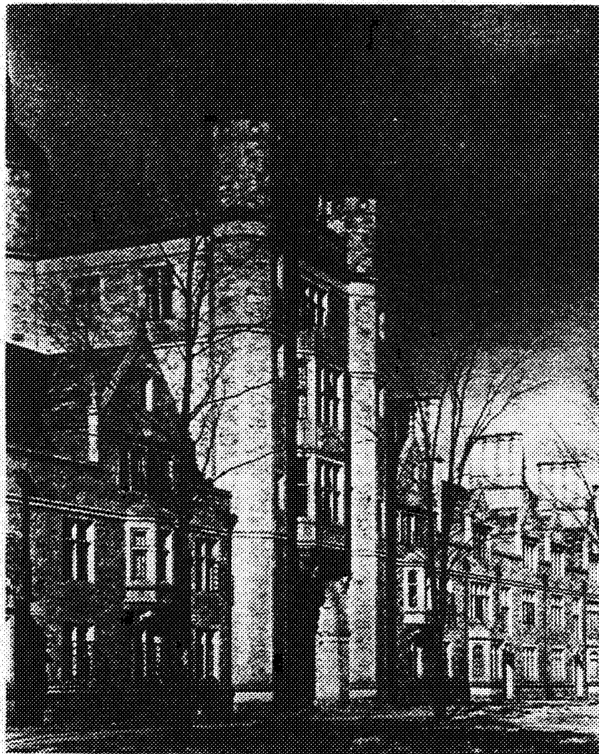
PLATE II. Central Arch, Lawyers Club Dormitory.
