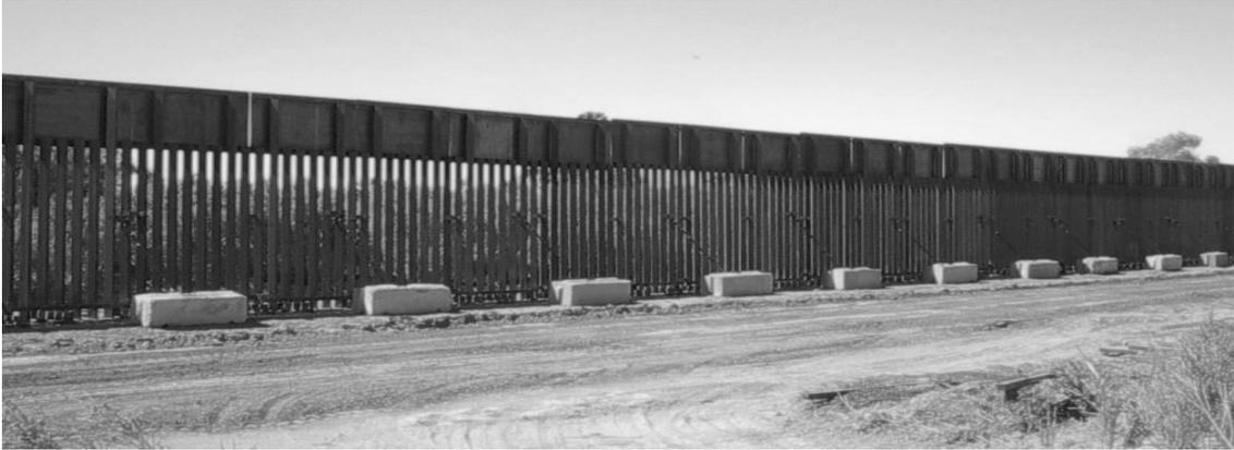
**Bollard Pedestrian Fence with Steel Sheath Extension**
