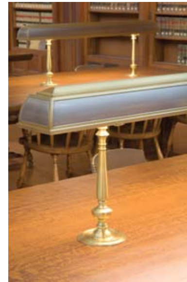
Brass table lights (left) are fitted with 28-W T5 lamps and linked to a daylight control system for reduced energy output. Now fitted with dedicated-socket, 18-W CFLs, the stack lights have a 20,000-hour life and better light distribution.
